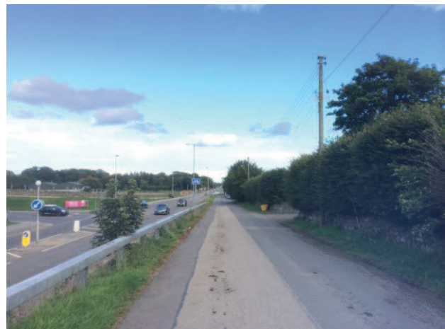
Access track is connected onto adjacent A944
