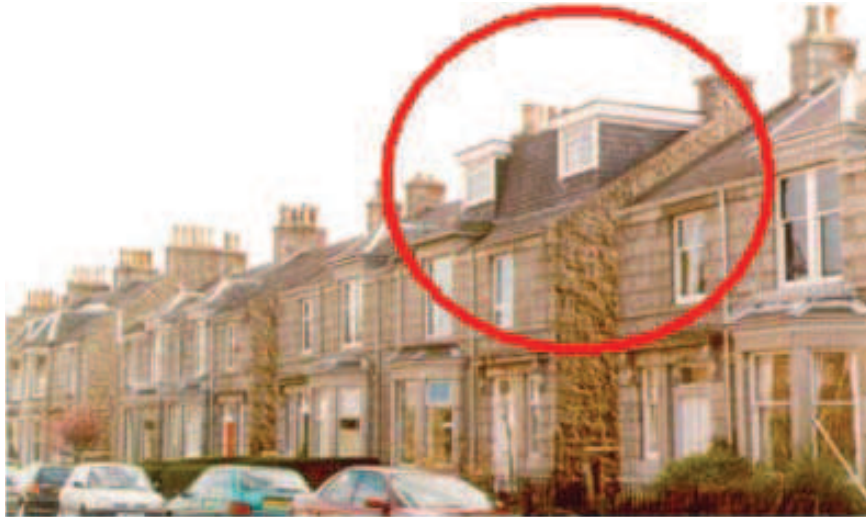
Example of a poorly designed roof extension – Dormers are too large, dominating the roof slope, and use of substantial infill panels and slated aprons contributes to bulky appearance
